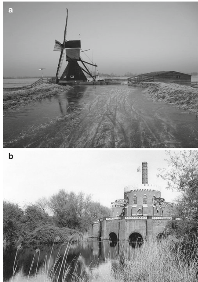
Fig. 4.7 (a) The Red Mill in Westlagelandspolder, now called the “Rode Polder,” was built in 1632. It is close to Leiden (in the village of Oud Ade) in the area where the first lakes were drained using windmills. The upper part of the mill, the house, can be turned and positioned with beams on the outside to be aligned with the wind direction. (b) The “Cruquius” was the first steam-powered pumping station in the Netherlands and was one of the three steam-powered stations built to drain the last and largest lake in the Netherlands, the Haarlemmer Meer, which was for many years a threat to nearby cities
